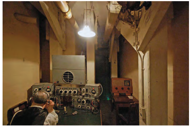
BBC OBA/8 outside broadcast equipment with 4-channel mixer central, monitor loudspeaker above, and at the sides power supply, peak programme meters, line drive amplifiers and ancillary cueing and talkback equipment (and a field telephone on the left)
